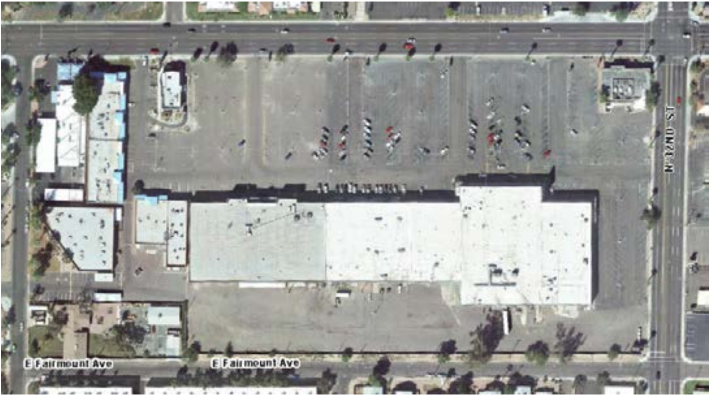
Aerial At The Time Of Purchase
